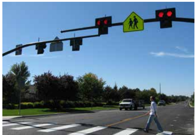
A HAWK pedestrian crossing signal could allow safe crossings in areas by Sarah Smith Elementary, or along Peachtree Dunwoody Road at Little Nancy Creek Park, for example.
