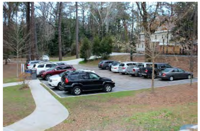
Newly resurfaced LNCP parking area with 17 defined spaces and improved entry/exit
