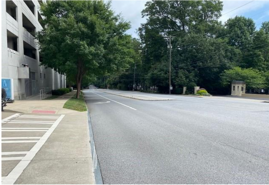
Comments: Site Driveway B looking north (Intersection 7).
