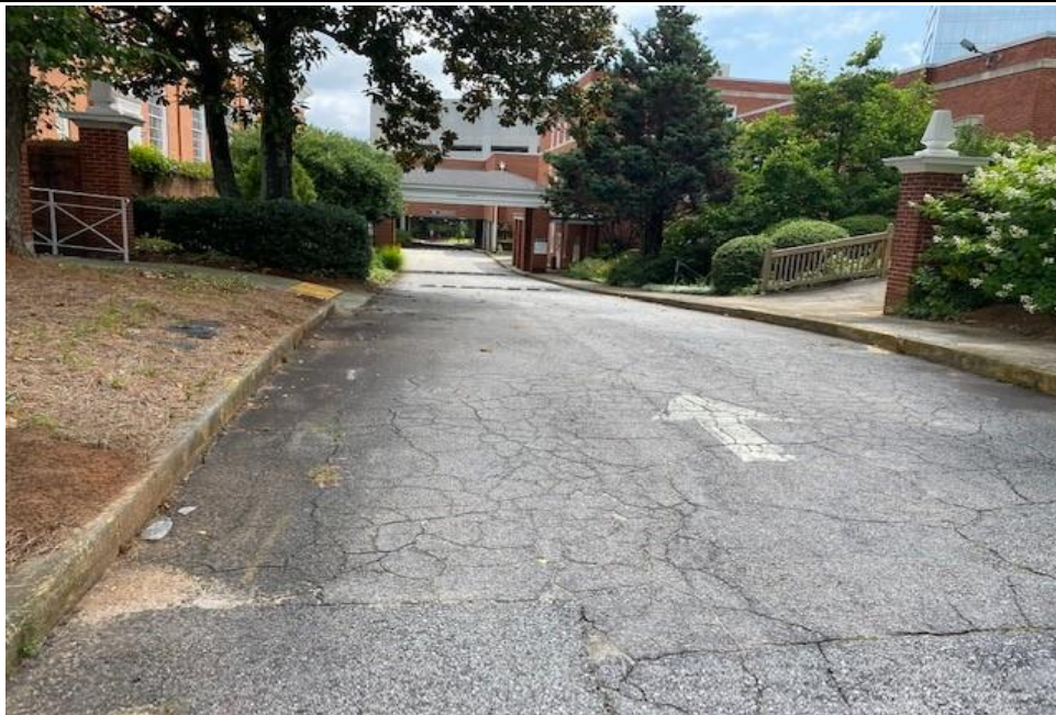
Comments: Site Driveway D looking east onto the site (Intersection 9).
