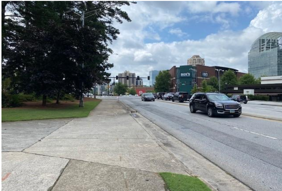
Comments: Proposed Site Driveway F looking south (Intersection 12).
